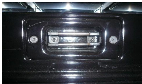
Figure No.17 - Accesses via which to clean the flue socket.
