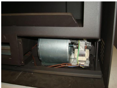
Figure No.11 - Electrical system
