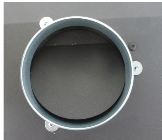
Figure No.9 - Correctly screwed nozzle at the 3 points with the washers
