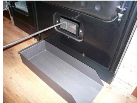
Figure No.18 - Accesses via which to clean the flue socket.
