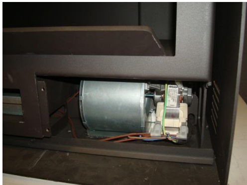
Figure No.5 - Electrical system
