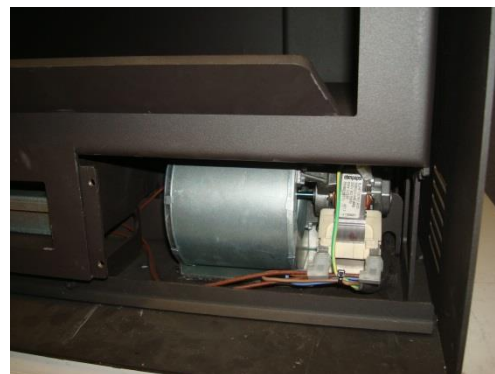
Figure No.6 - Electrical system
