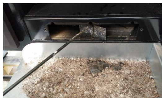
Figure No.22 - Accesses via which to clean the flue socket.
