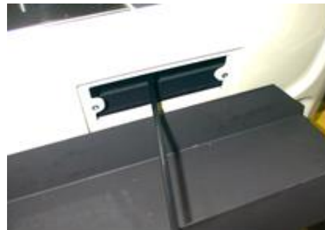
Figure No.19 - Accesses via which to clean the flue socket
